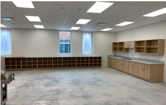
Casework is installed in the art rooms 03/11/2023
