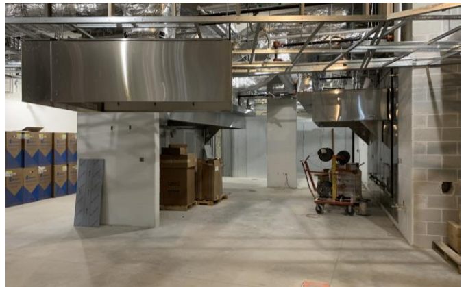
Kitchen hoods are installed 03/11/2023
