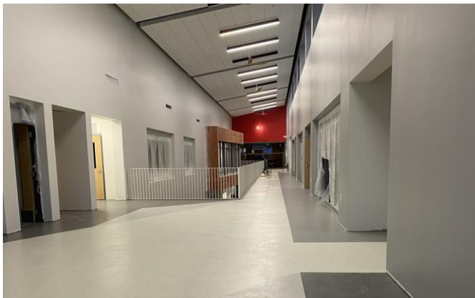
Rubber flooring and ceiling tile installed in the main entry corridor 03/30/2023
