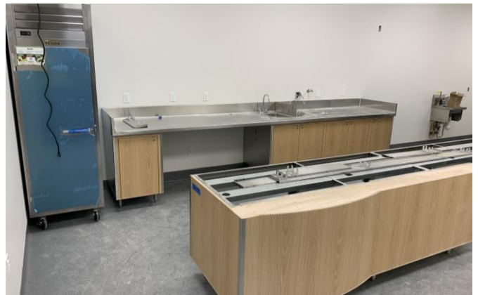
Kitchen equipment gets installed in the satellite serveries 03/11/2023
