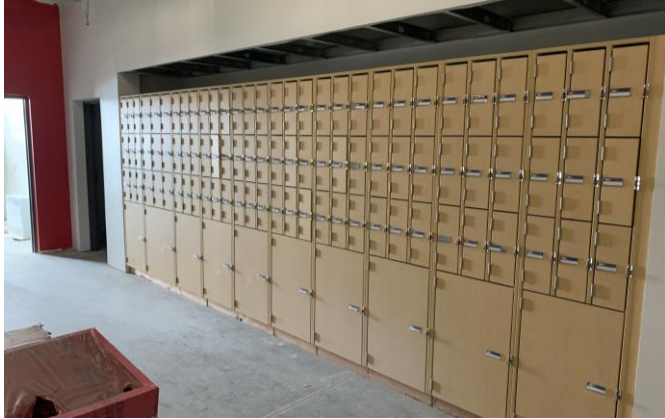
Completed music casework 03/11/2023
