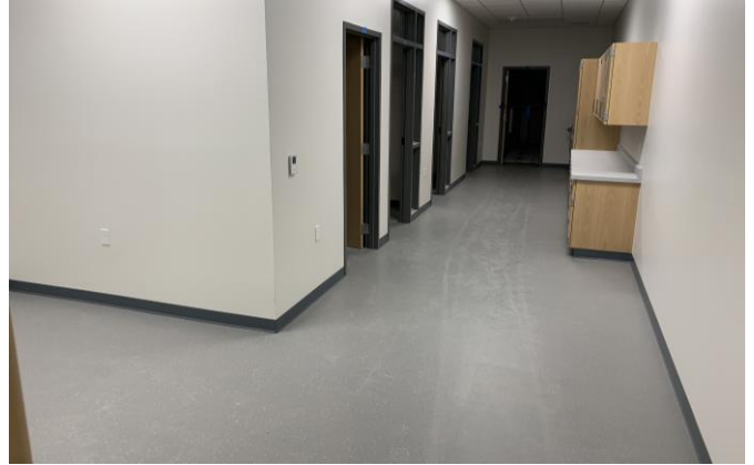
Completed rubber flooring in the health/nurse room 03/11/2023
