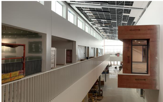
The main entry corridor receives paint and ceiling grid 03/11/2023
