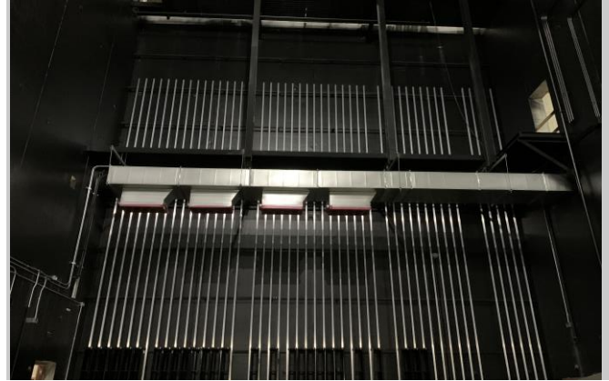
Theater rigging in the auditorium has started 03/11/2023
